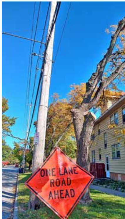
Vancuren working along Fulton Road. There are two tiers of four wires each. The top ones are the responsibility of tree trimming crew.
