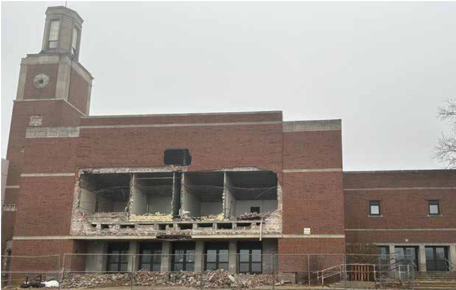
Parma Senior High School Demolition
