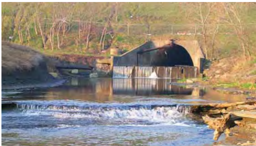
Six foot concrete fish barrier and eroded stream bank on West Creek at I-480 before restoration.
